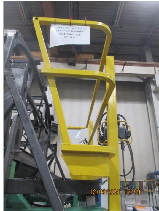
Improved Fall Protection
