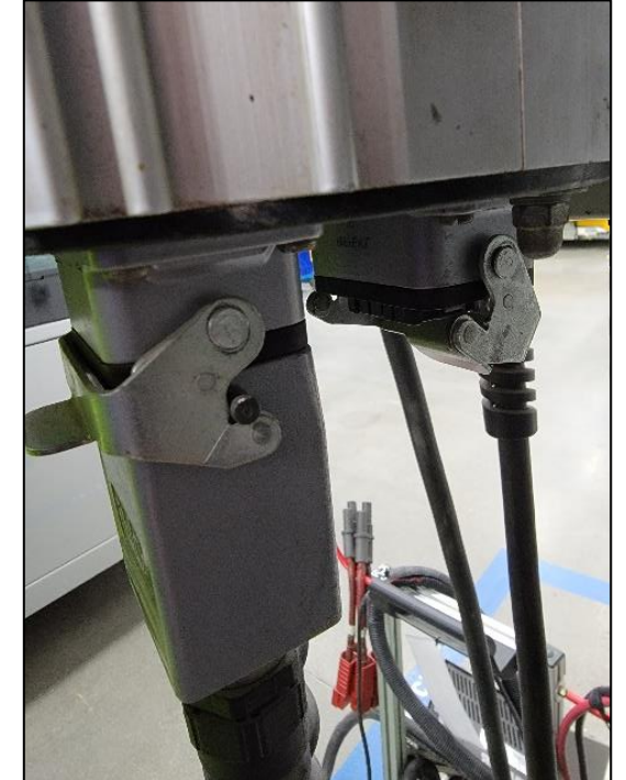
Fixed Broken Lock on Bus Lift
